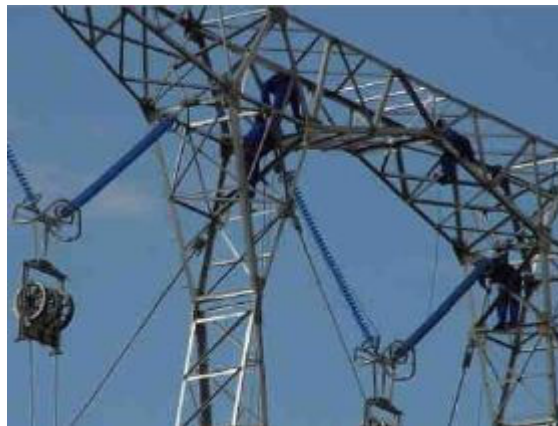
Using pulleys to hoist cable
