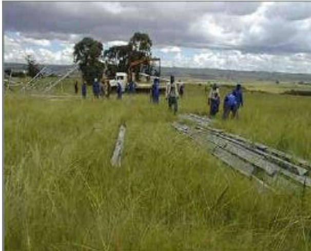
Steel delivered for assembly
