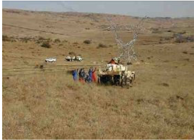
Stringing pilot cable with pilot tractor
