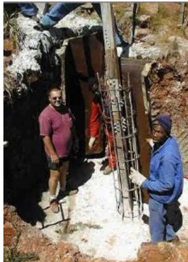
Foundation steelwork
