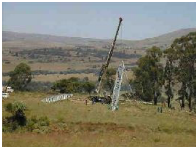
Raising the pylon
